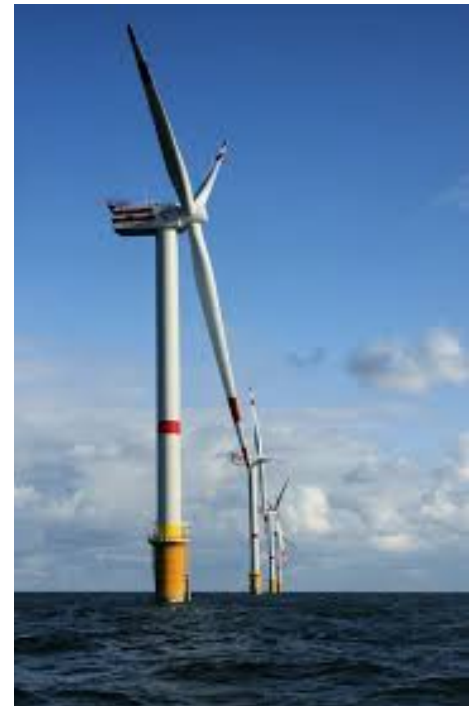
Figure 6.3: An off shore Wind Turbine
